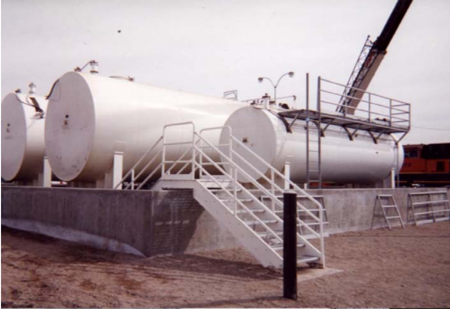
Two 30,000 gallon and one 5,000 gallon UL142 tanks on saddles.
